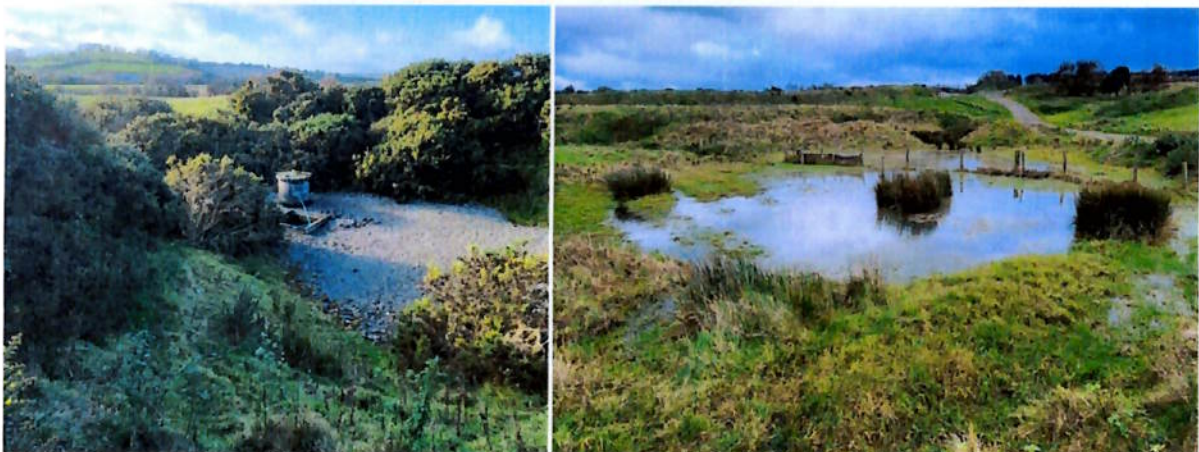
Figure 4-6 - Infrastructure at the source of the 'spring' (left) and example of FL4 downhill (right)
